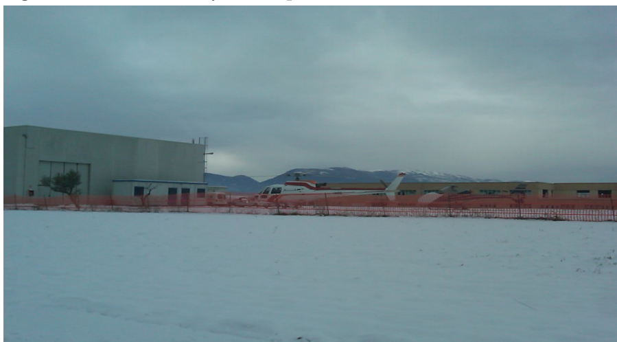
Figure II.1 - Finbox facility and heliport
